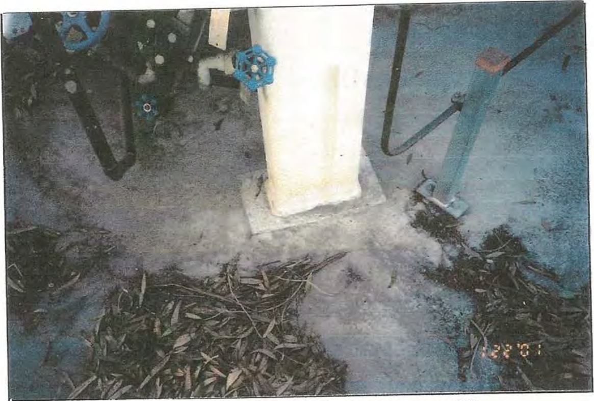
Auxiliary Oxygen Tank Anchorage C2
