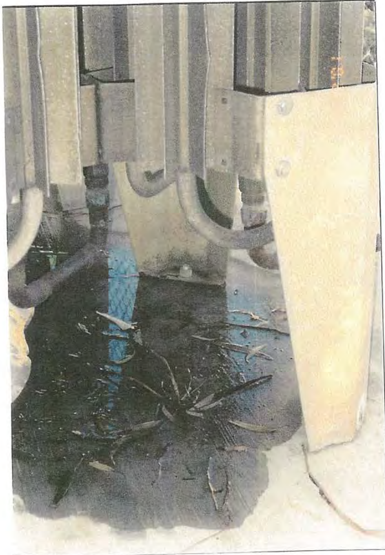
Auxiliary Oxygen Tank Anchorage C2
