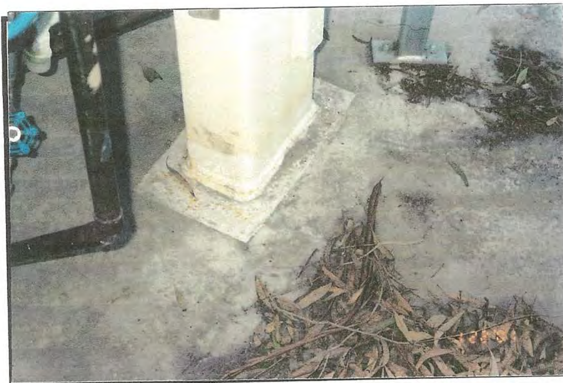
Auxiliary Oxygen Tank Anchorage C2
